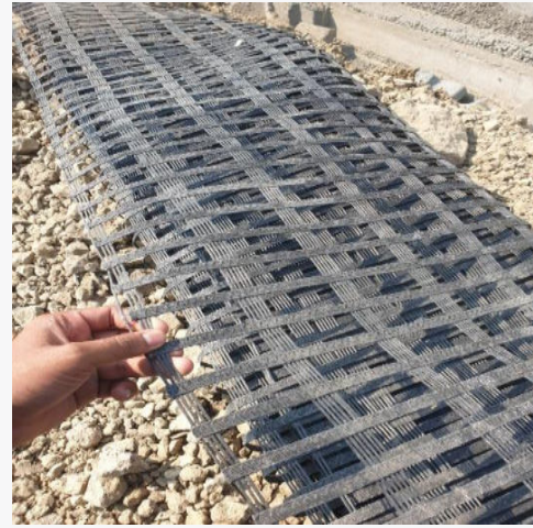
Fig. 4 Geo-textile (PF) in road construction
