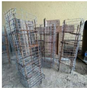
Fig.2: Reinforcement On CRC1
