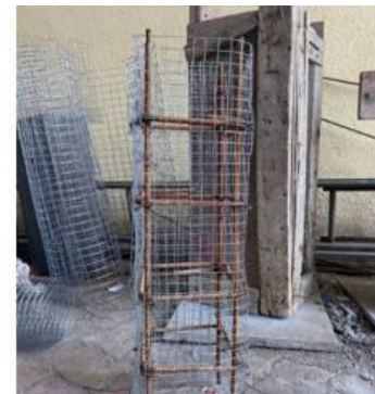
Fig.3 Reinforcement On CRC2 (Welded Iron Mesh)
