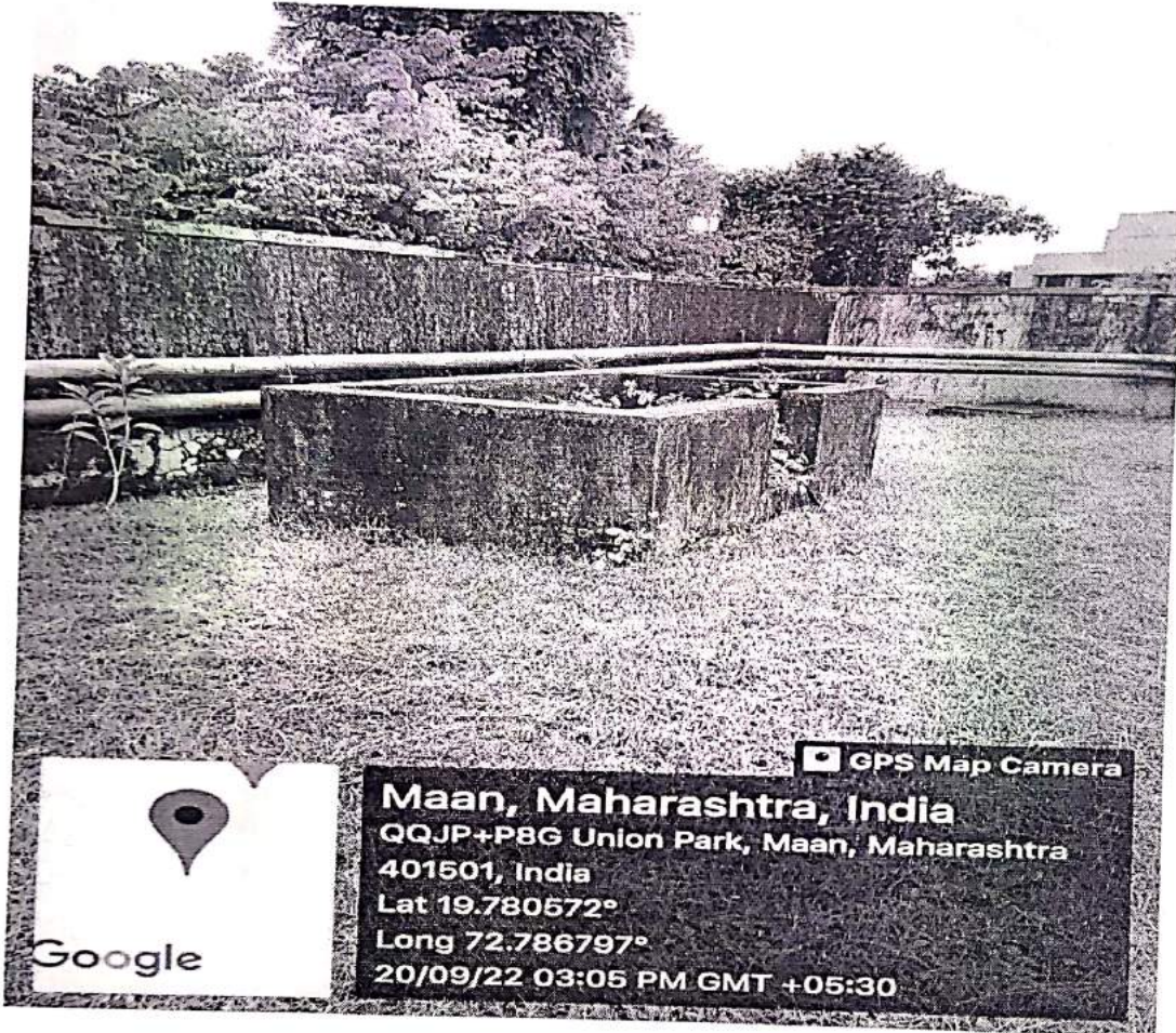
Solid Waste Disposal
